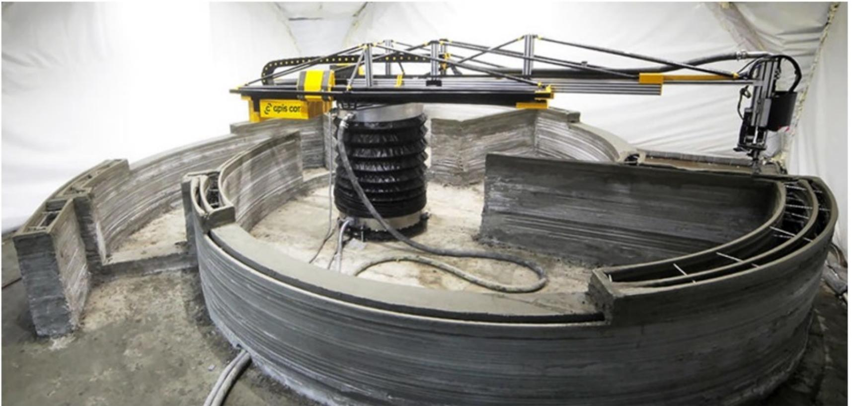
*(fig 4.2.1) This picture illustrates how a 3D printer with a main expandable pylon could build the structure without having to move any of its parts except for the robotic arm.*
